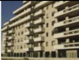
Apartment block (1 riser) independent speaker between backbones and risers
